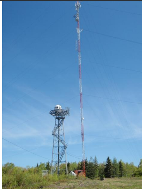
NSDNR Fire Tower, immediately west of the Project Site and Turbine 3 location.
